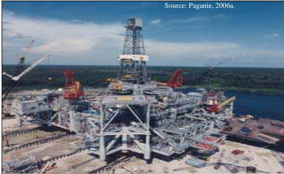
**Figure 10. Independence Hub's topsides under construction at fabrication yard near Corpus Christi, Texas.**
